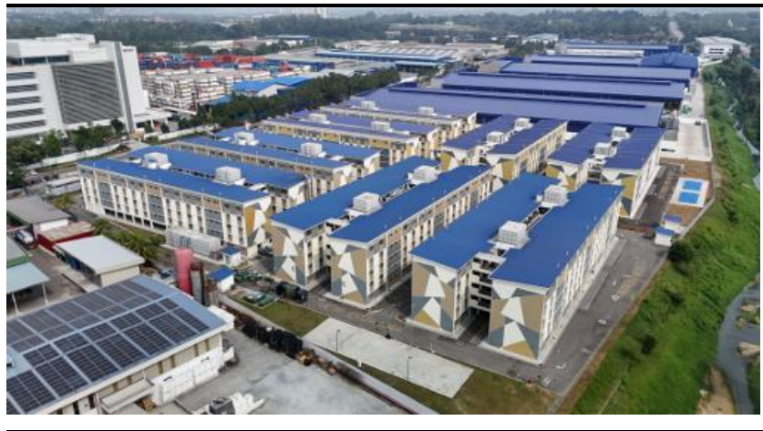
Fig 1: Worker accommodation asset in Pasir Gudang, Johor
