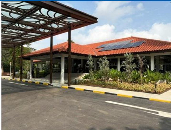
Figure 3: CRC entrance with solar panel roof tops
