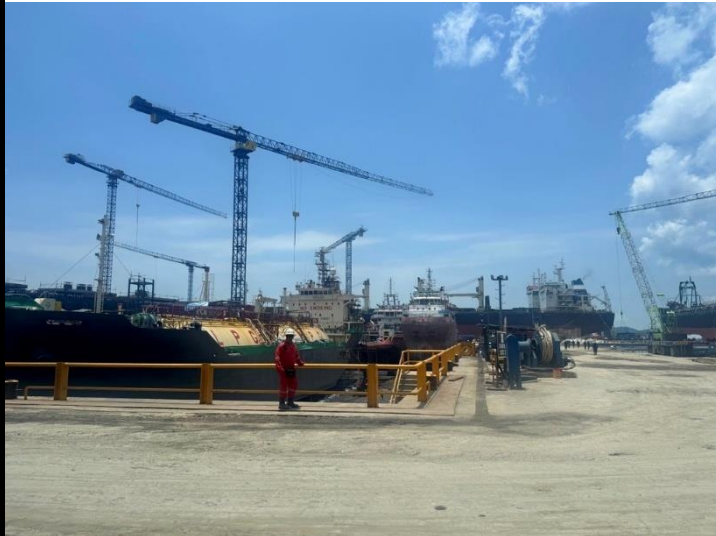
Figure 3: MPM's yards busy with repair jobs
