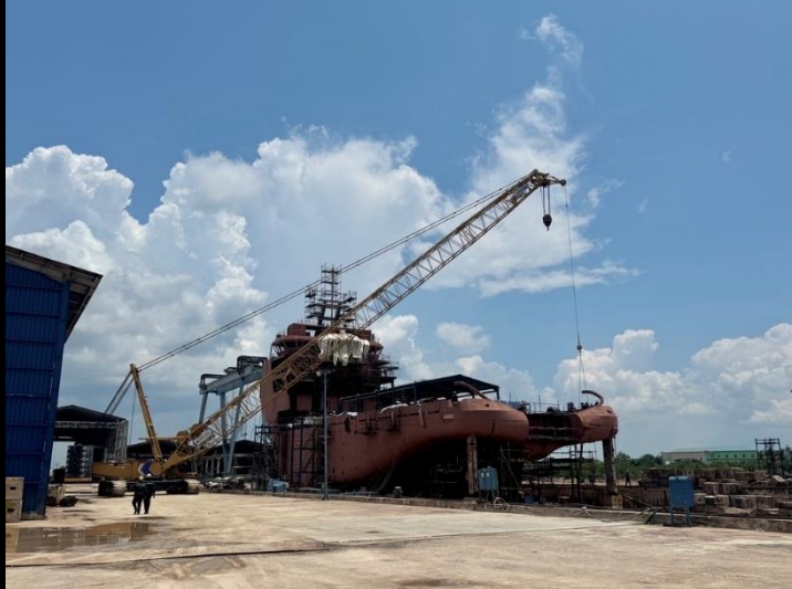
Figure 1: Construction of AHTS 2 at MPM's Batam yard
