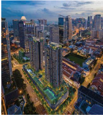
Midtown Modern Client: MTG Apartments Pte Ltd & MTG Retail Pte Ltd Approx Contract Value: S$227.5 million
