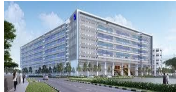
JTC Space @ Ang Mo Kio Street Client: JTC Corporation Approx Contract Value: S$287.5 million
