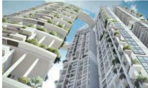
One Pearl Bank Client: ARECA Investment Pte Ltd Approx Contract Value: S$190.0 million
