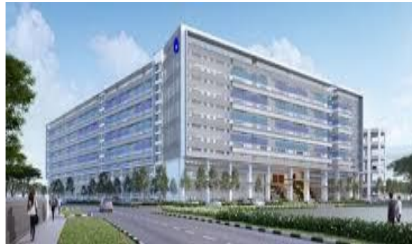
JTC Space @ Ang Mo Kio Client: Tiong Seng Contractors Pte Ltd
