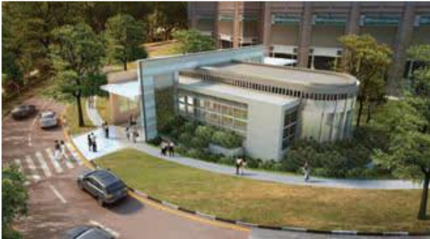
Contract T220 – Great World Station Client: Land Transport Authority Approx Contract Value: S$315.9 mil
