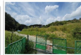
← Site of Otawara Solar Power Plant
