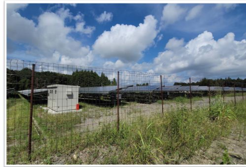
↑ Kami Ishikawa Solar Power Plant
