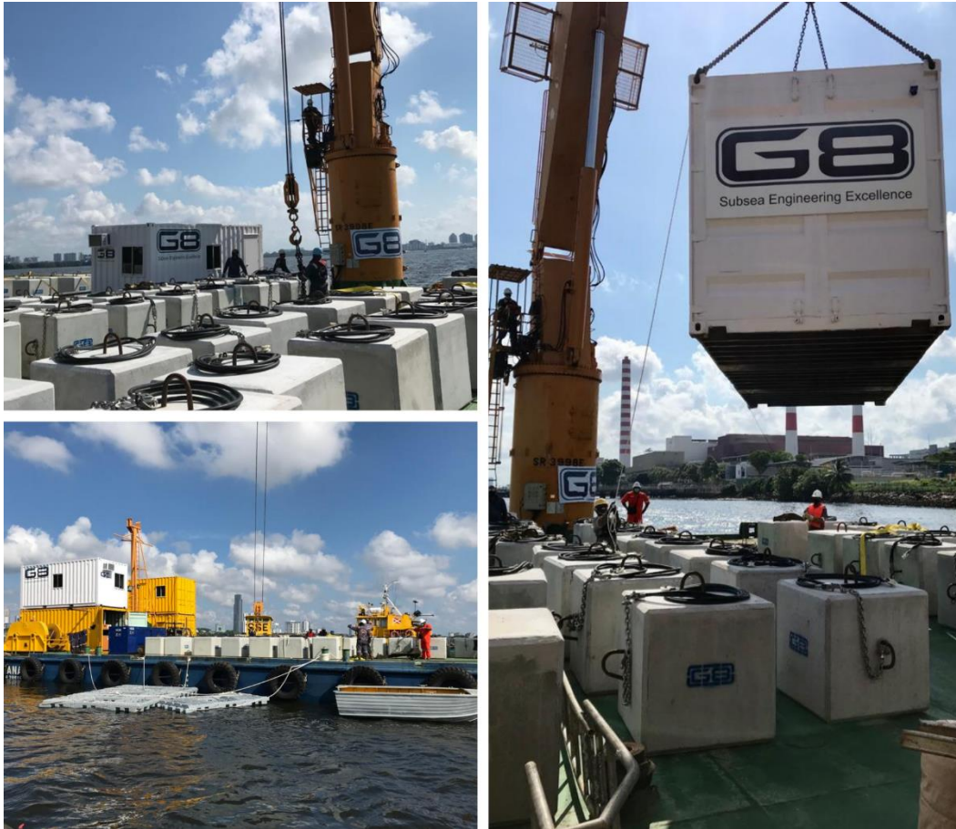
G8 installing underwater mooring system for floating solar
