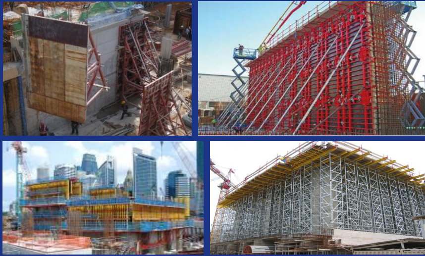
Advanced Formwork System
