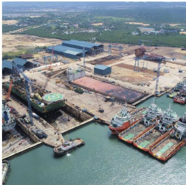
Figure 6: Extension of dry dock 1 from 150m to 240m, completed on 15 Feb 2022
